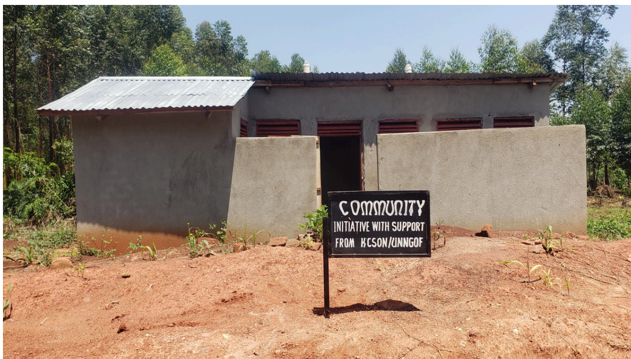
Fig. 2: A newly constructed five stance pit latrine at Ruzaire Primary School, built through the collective efforts of the community and the Kitara Civil Society Network.
