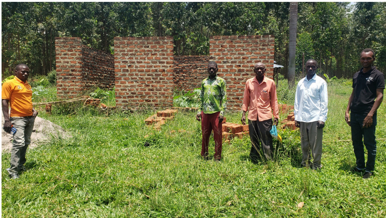
Fig 3: A new office block under construction at Ruzaire Primary School.
