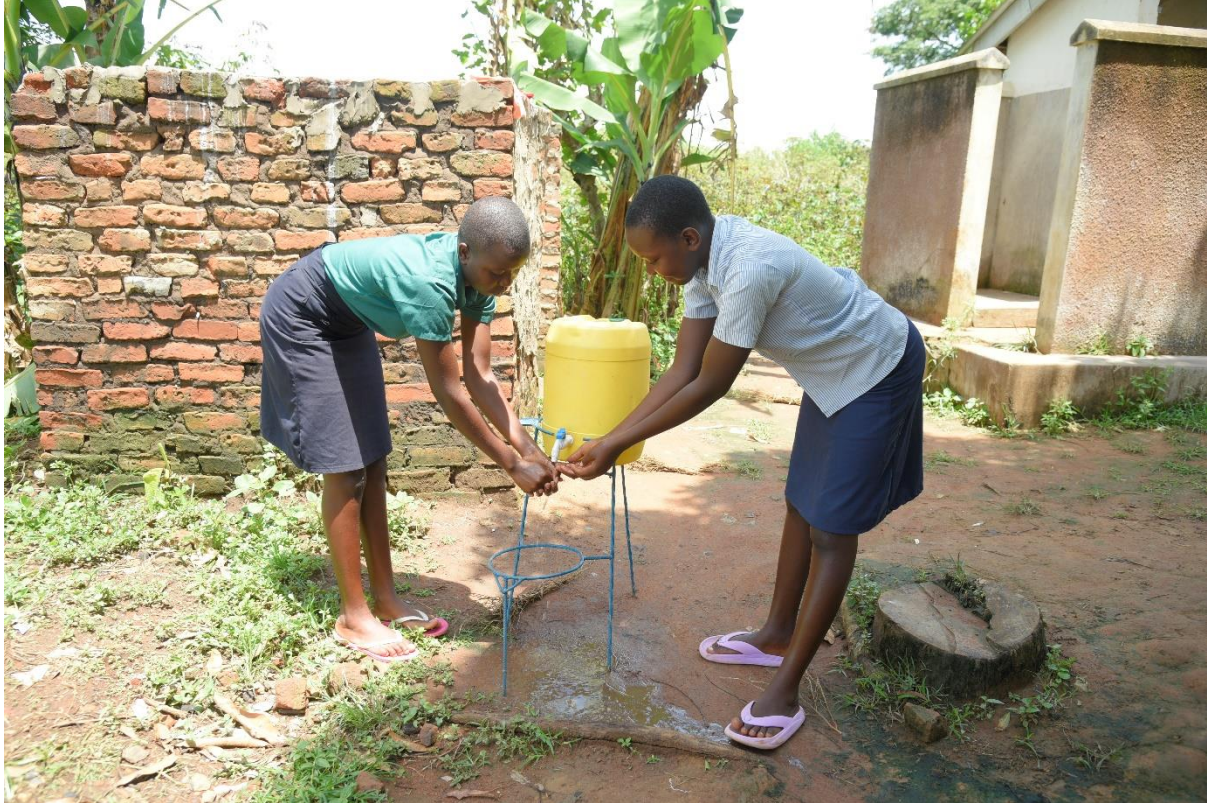
Fig 2: Pupils at Nambiri Primary School using one of the newly acquired handwashing facility on 22 nd October 2024.
