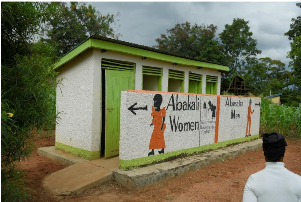
Fig 2: A photo (taken on 23rd October 2024) capturing the newly constructed pit latrine and adjacent bathroom at Nabuli Health Facility, designed to improve sanitation and comfort for in-patients. This upgrade reflects ongoing efforts to enhance healthcare infrastructure and meet the needs of the community.
