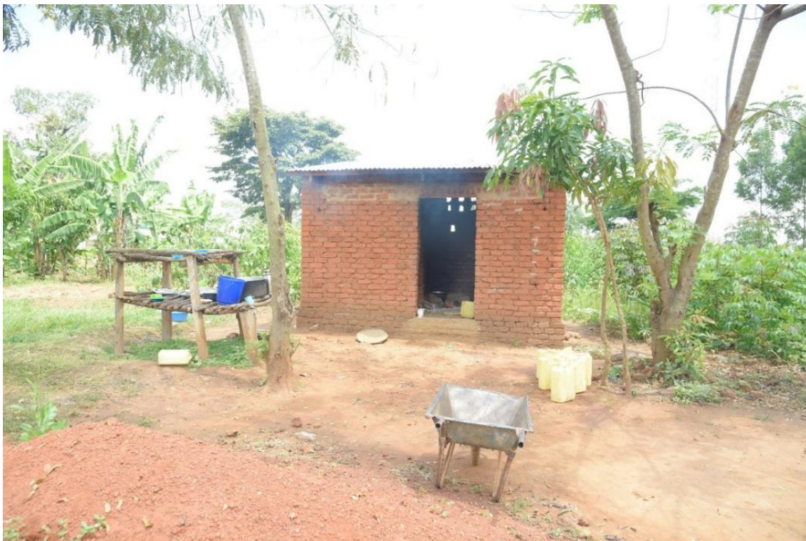
Fig.3: Newly built kitchen for teachers at Kameruka Primary School as captured on 22 nd October 2024
